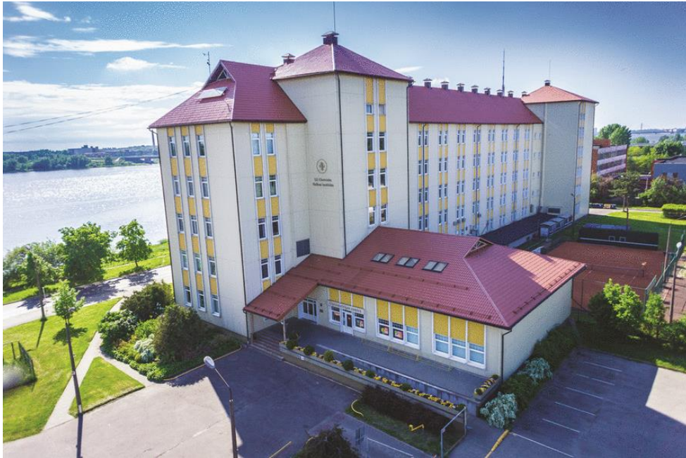
ISSP UL building in 2012 (Photo by A. Zavadskis)
